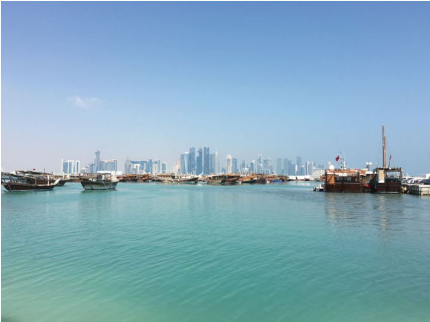
Fig. 2.3 Skyline of Doha's West Bay
